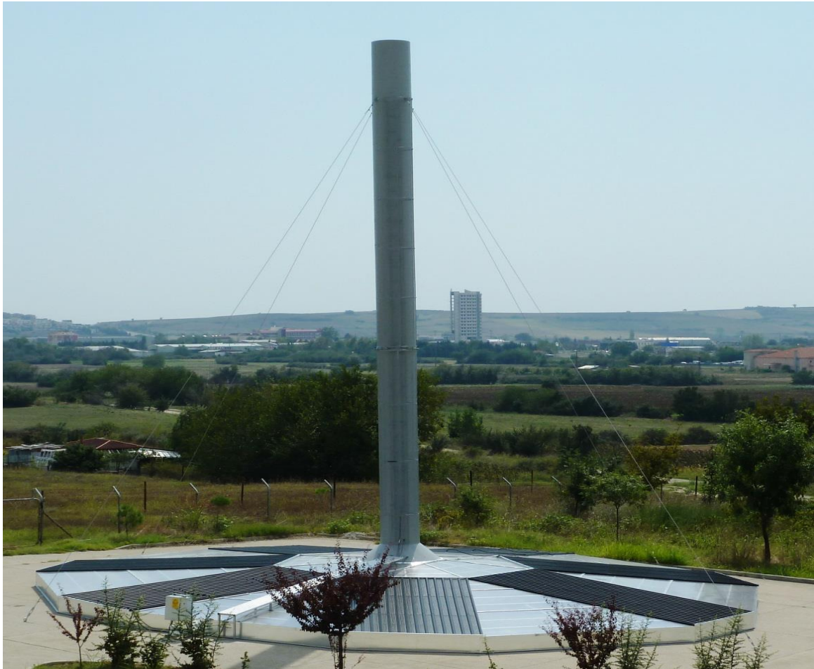
Figure 2. Hybrid Solar Updraft Tower Test Unit
